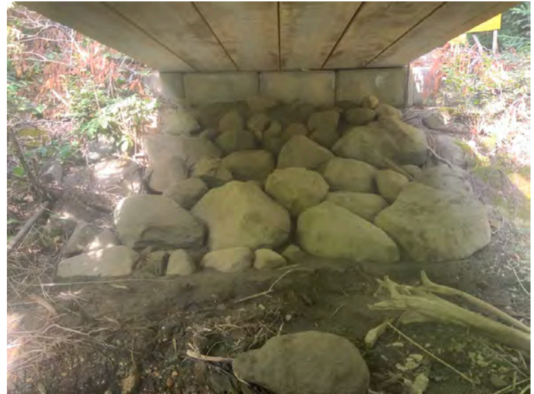
Left Bank Abutment when facing downstream
