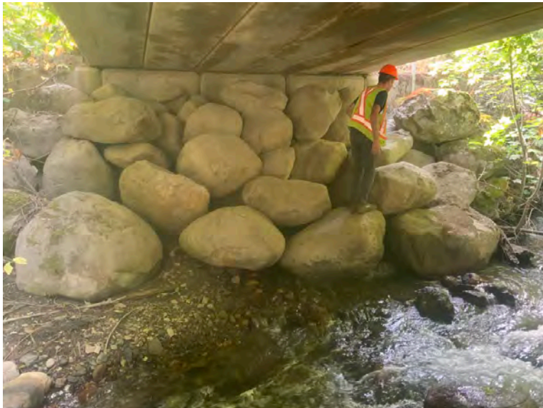
Right Bank Abutment when facing downstream
