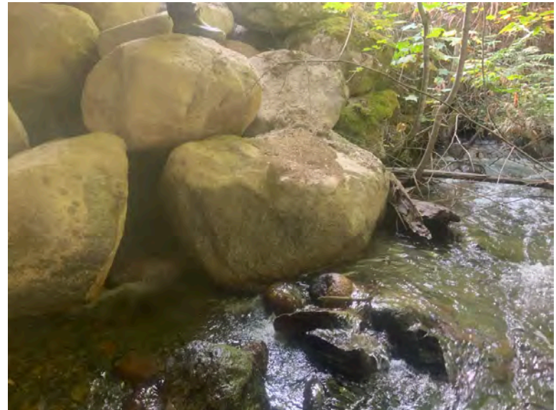
Right Bank Abutment when facing downstream
