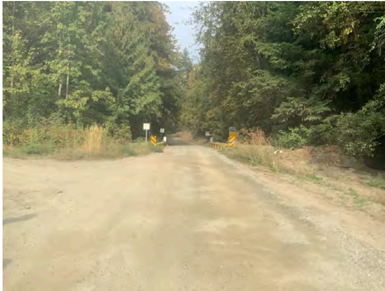
Approach from Right Bank when facing downstream
